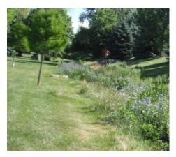
*Bioswales work to filter out stormwater pollutants.*
